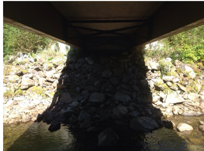
Right Bank Abutment when facing downstream
