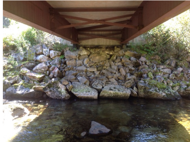
Left Bank Abutment when facing downstream
